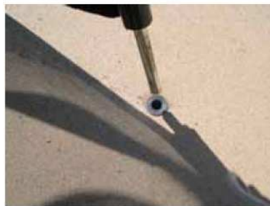
Fig. 5. Fixing the anchor into the ground
