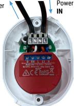
Connect the power (input and output) cables, as shown on the picture above.
